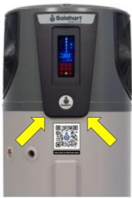
Pop the Display Panel off its mount by pulling firmly on the bottom corner(s)
