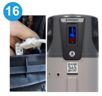
Fully **insert and latch** the Display Module Module **cable** and re-mount the Module on the water heater.
