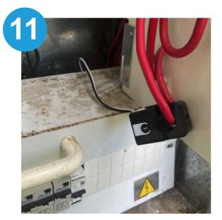
At the switchboard, clip a CT onto the water heater supply wire for power monitoring (with the arrow pointing towards the water heater)
