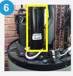
Remove the Top Cover from the water heater and locate the Heat Pump Controller module
