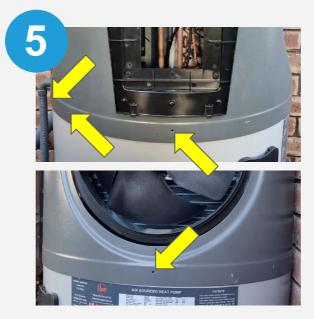
Remove all screws securing the Top Cover onto the heater jacket
