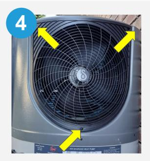
Remove both fan covers by removing the three screws and pulling away from the heater
