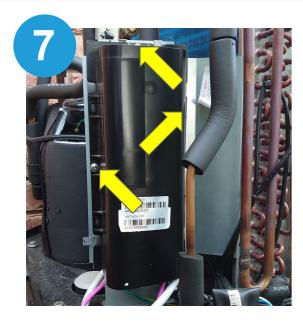
Remove the screws holding the Heat Pump Controller cover in place to expose the Controller board
