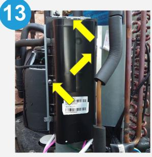
Re-mount the water heater Controller cover and screws
